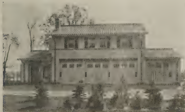
Garage of Everett L. Brown, in the basement of which water supply system is installed
